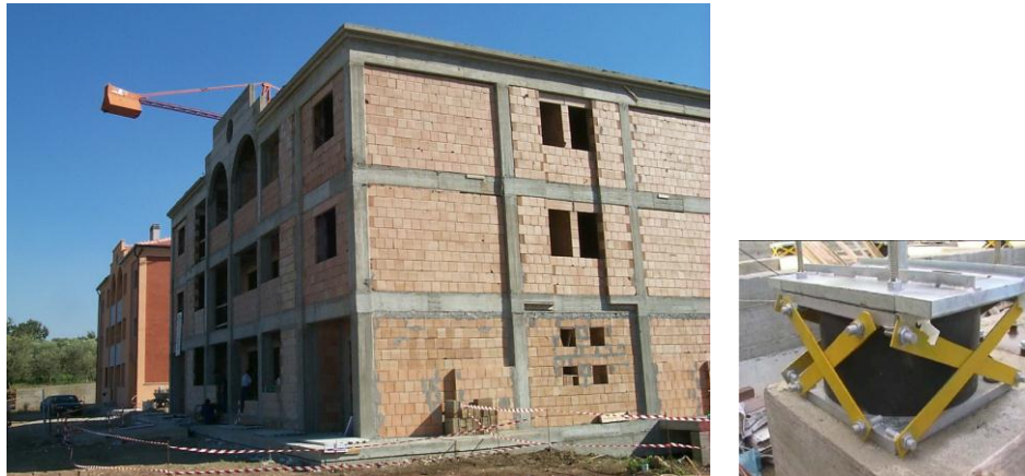
Figure 1.10 Three-story base isolated building with special mixed bearings (HDRB + Slider), Rapolla, Italy
