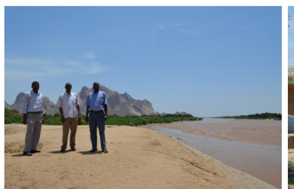
Plate 9: View of the Gash Protection embankment
