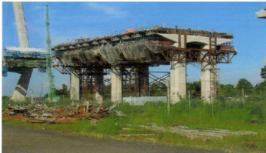
Fig.13 Construction view before collapse
