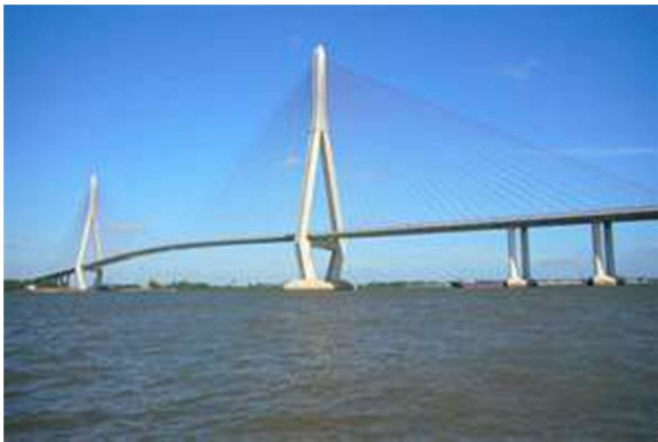
Fig.19 Can Tho Bridge after completion
