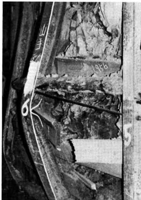
Photo 10.4 The State of Yielded H-125 Steel Ribs at STA. 33 km, 220 m.
