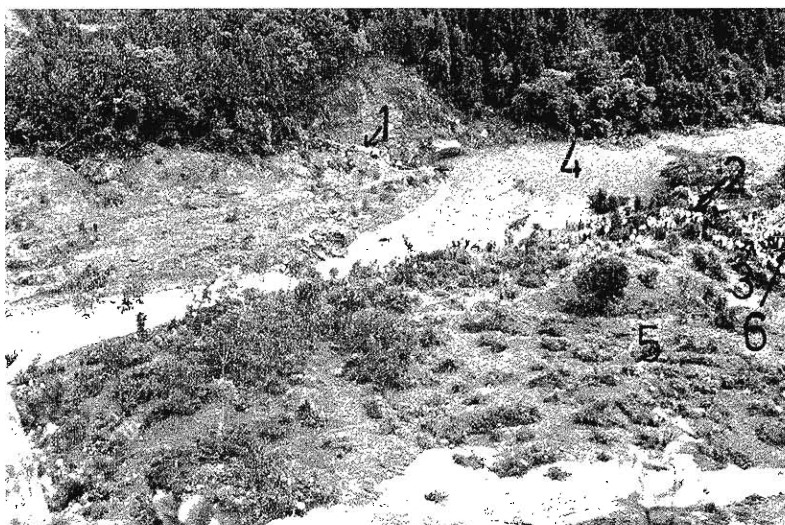
Photo 2. The lower part of Shigeto landslide area.
