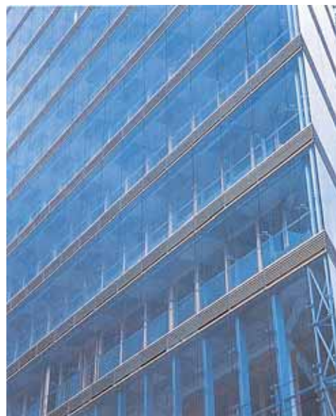
Photo 1 Storey high double skin glazing facade
