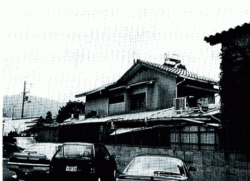
Photo 13 Tested House TA.
