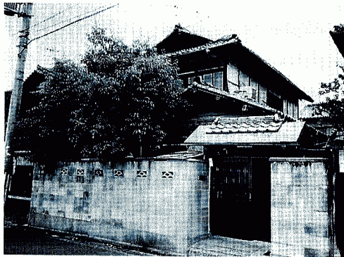
Photo 7 Tested House SI.
