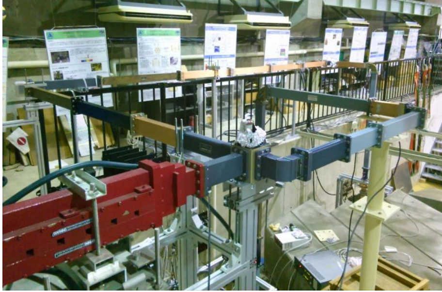
Figure 2.11: Waveguide after rearrangement, the waveguide switch (at the center of the figure) was installed downstream RF circulator (red) for the switching operation between the 4.5 cells thermionic cathode RF-gun and the photocathode RF-gun.
