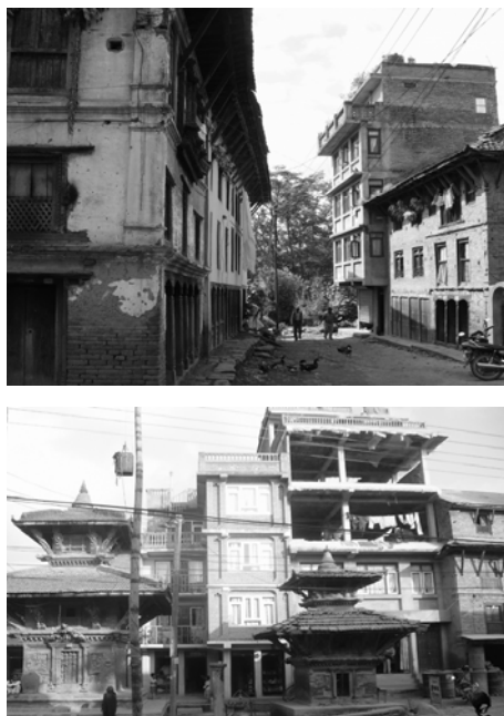
Fig.2 Unsafe modern houses along with indigenous houses.
