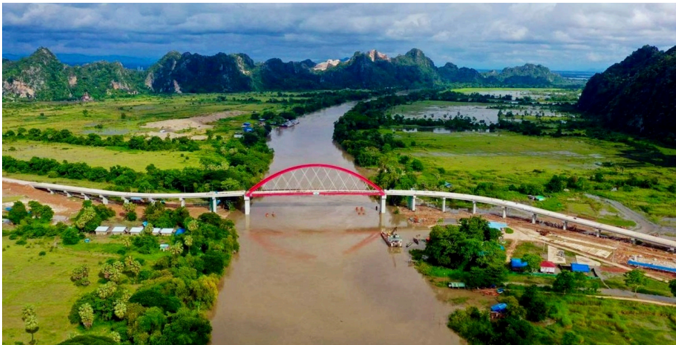
Tham Malay Bridge near Kyaik Maraw, Mon State, Myanmar. Photo: Wikipedia Commons
