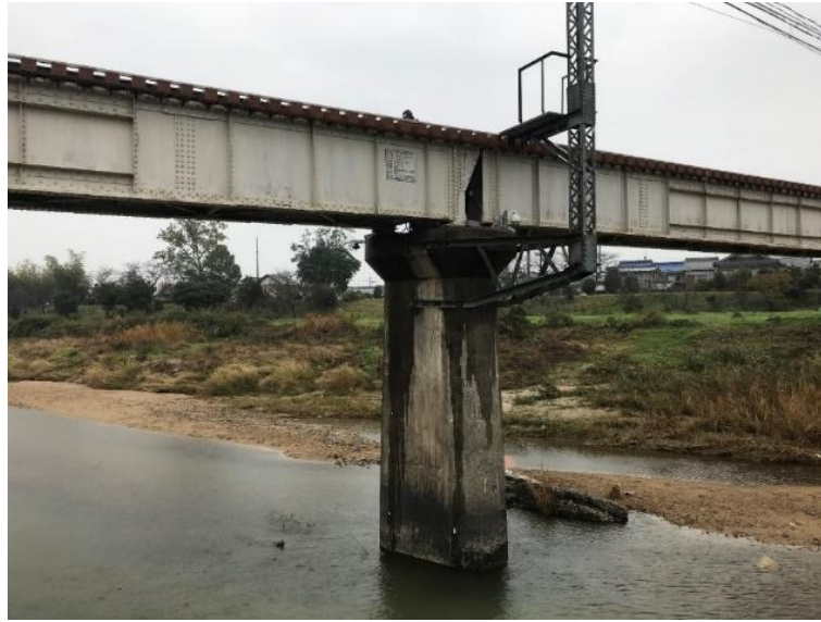
Figure 2.10 Monitoring pier of the railway bridge.
