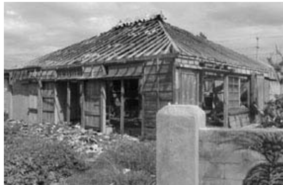
Photo 5. Completely destroyed wooden house.
