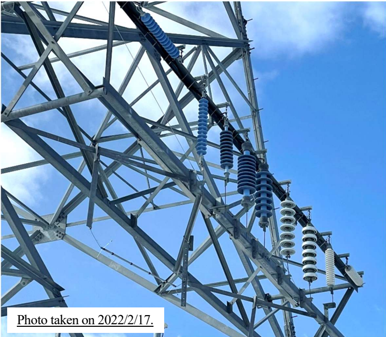
(c) Insulators for snow accretion observation ( h = 10\text{ m} )
