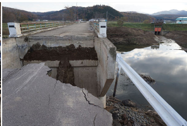
(b) Futohoro Bridge over Tokoro River
