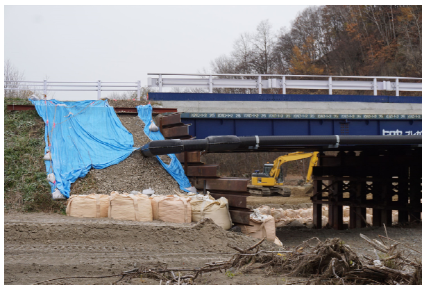
(a) Kiyomi Bridge over Tokoro River
