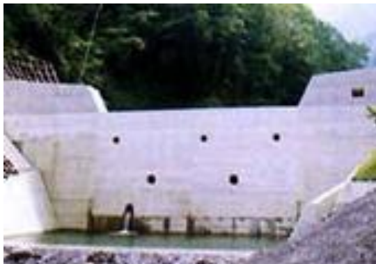
Fig. 3 Closed-type sabo dam
