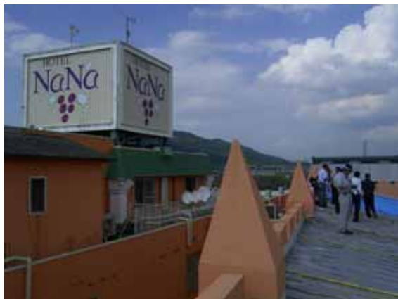
Photo 5 Damaged roof (Right) and control building (left).
