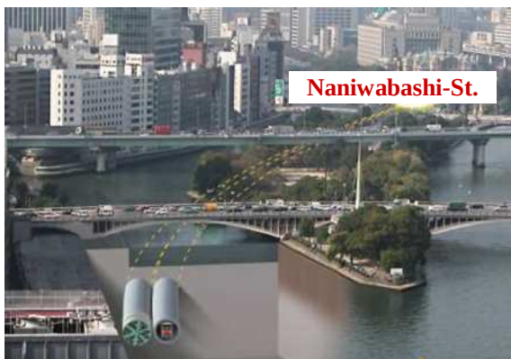
Photo. 1 Shield tunnel under the River Tosabori
