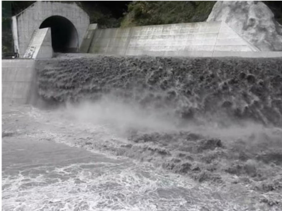
Figure 10: Operational view of the Koshibu SBT outlet.
