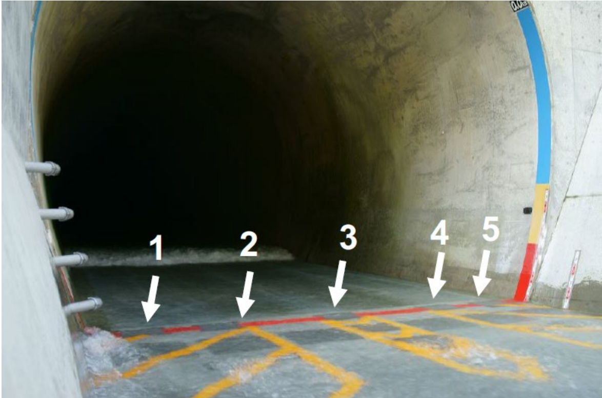
Figure 18: Koshiu Dam SBT outlet with five IPs installed. White arrows indicate the impact plates, from (Koshiu & Sumi, 2020).
