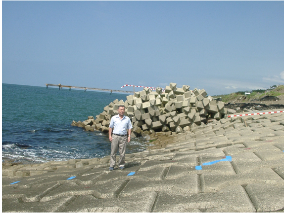
Fig. 20 A view of recently constructed erosion-protection work on Ogata coast, with the observation pier standing in the background
