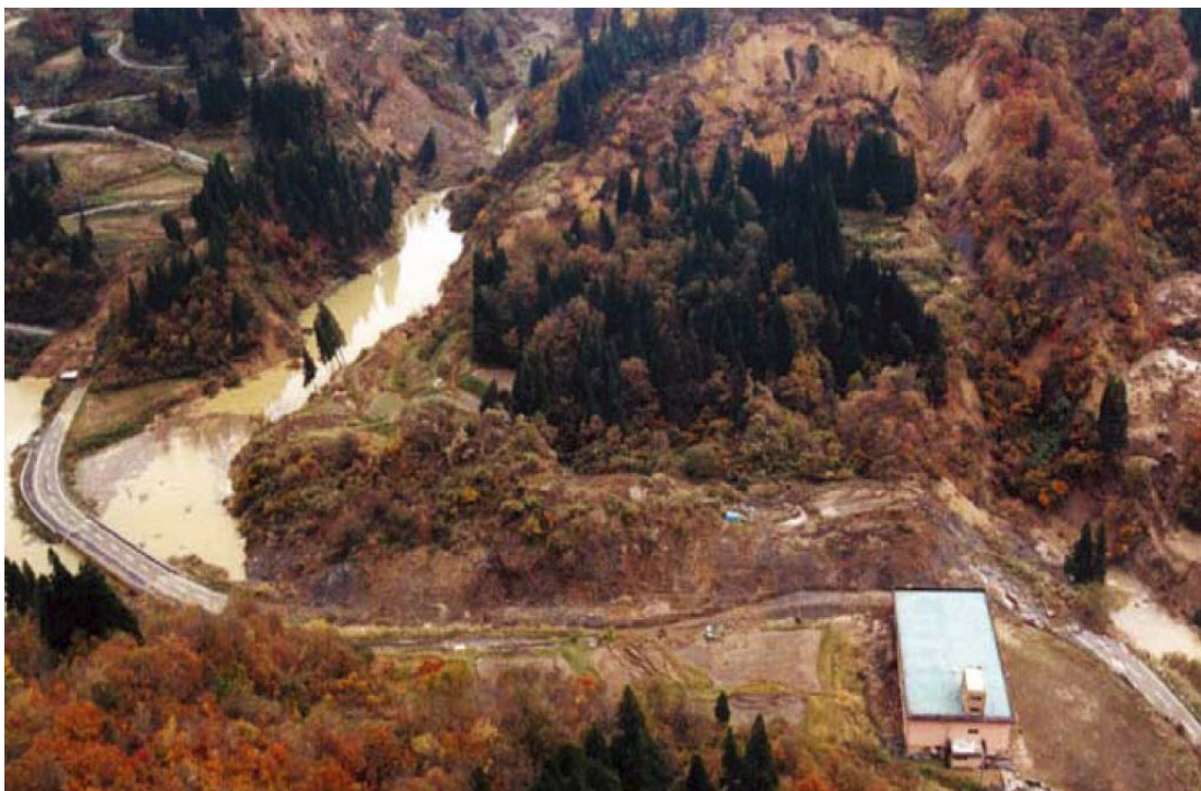
Front view of the Higashi-Takezawa Landslide
