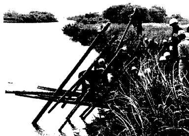
Photo 2 Kawakura in the Jintsu River (during a flood fighting drill)
