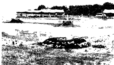
Photo 7 Kamadan ko(circular hooping by sandbags) in the Yodo River (during a flood fighting drill)
