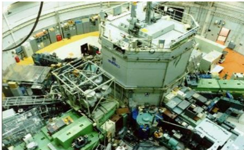
Fig.2-4 Kyoto University Research Reactor.
