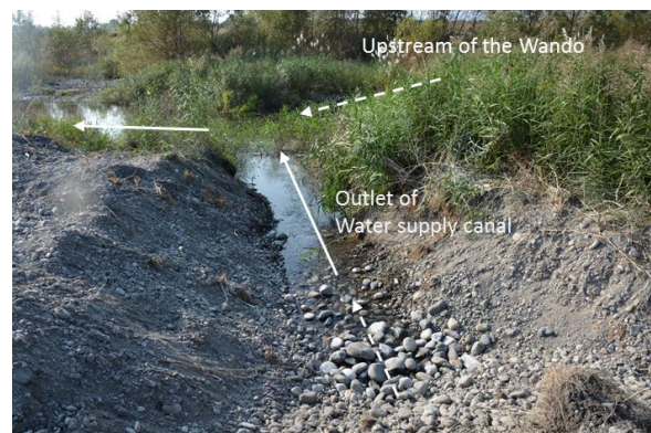
Fig. 11 Landscape of upstream of the Wando
