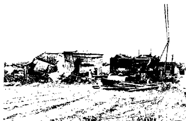
Photo. 10. Damage to a concrete block house.
