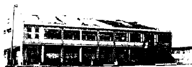
Photo. 12. Damage to Watomari junior high school.
