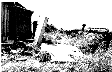
Photo. 23. Failure of concrete block fence.
