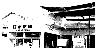
Photo. 22. Roof failure due to uplift.
