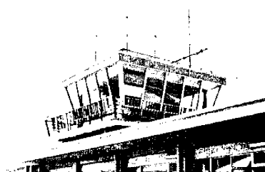
Photo. 16. Damage to the control tower in Okinocrabu.
