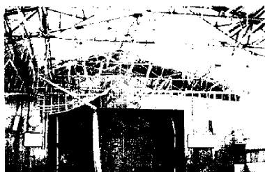
Photo. 13. Roof failures of Watomari junior high school.
