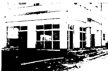
Photo. 18. Damage to glass panes in Tamina.
