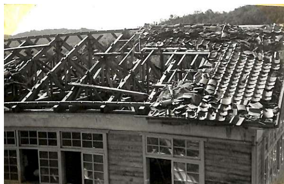
Photo 1. Damage to clay tile roof of low-rise timber building caused by strong wind during typhoon Vera (1959) from DPRI-KU archive.
