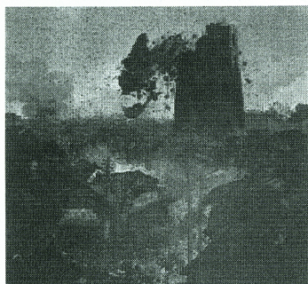
Photo 5 The brick construction structure which collapsed by the great Kanto Earthquake in 1923, described in the old postcard
