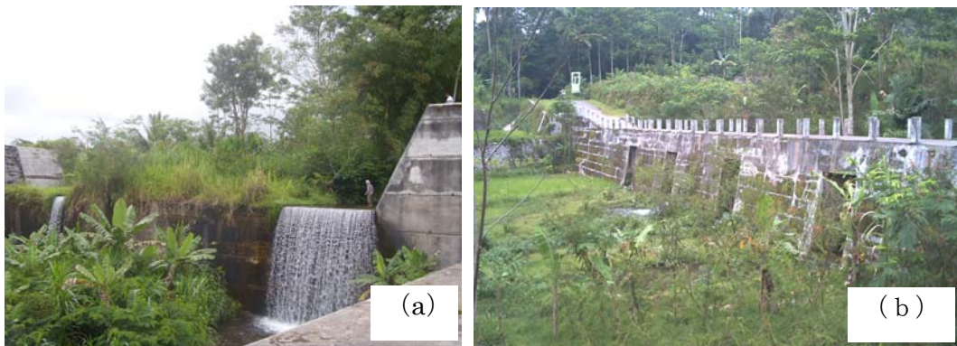
Photo 3.3 Existing of sabo works on slopes of Mount Merapi. (a) A Check dam functioned as an intake and a sand pocket on Blongkeng River (BLD1). (b) A Consolidation dam on Putih River functioned as a bridge (PU-C8A) (Photos were taken in December 2008)
