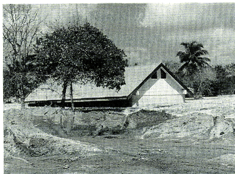
Photo 1. Damaged house by Lahar
