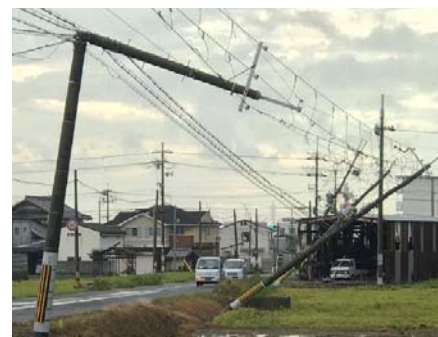
Fig.53 damage to telephone pole (科研費報告書, 2019)
