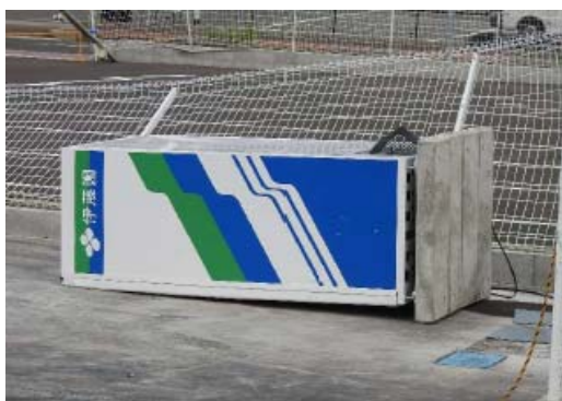
Fig.34 toppled down vending machine (科研費報告書, 2019)
