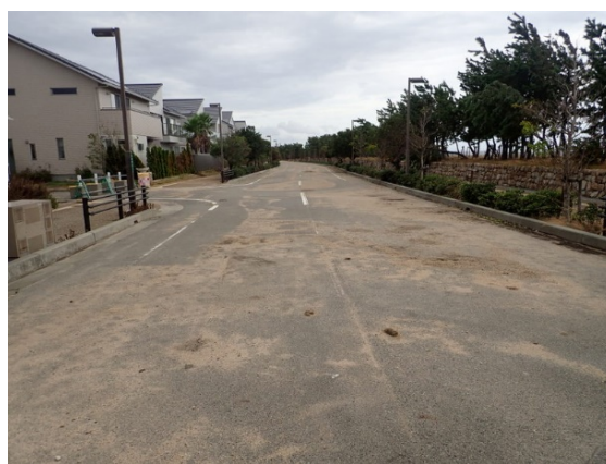
Fig.56 Trapped sands by wave overtopping at Ryofu-cho in Ashiya (科研費報告書, 2019)
