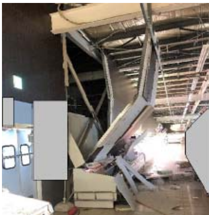
Fig.28 damaged to a store partition wall (科研費報告書, 2019)
