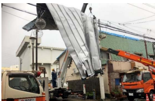
Fig.35 damage due to scattered steel sheet roof (科研費報告書, 2019)
