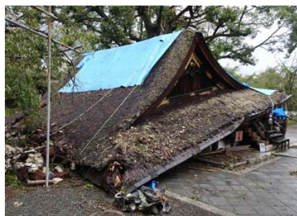
Fig.38 collapse of a Shinto shrine (科研費報告書, 2019)
