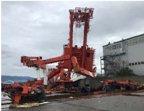
Fig.49 gantry crane collapse (科研費報告書, 2019)
