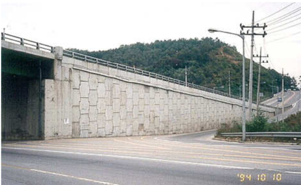
Fig 3.4 Reinforced approach embankment for overpass bridge, Kyeongchung Highway.
