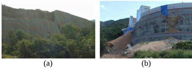
Figure 5.3 Total failure of entire reinforced earth wall ((a) Highway construction site - Overall sliding failure; (b) High school construction site - Overall sliding failure and facing block sliding)(Lee and Cho, 2011)
