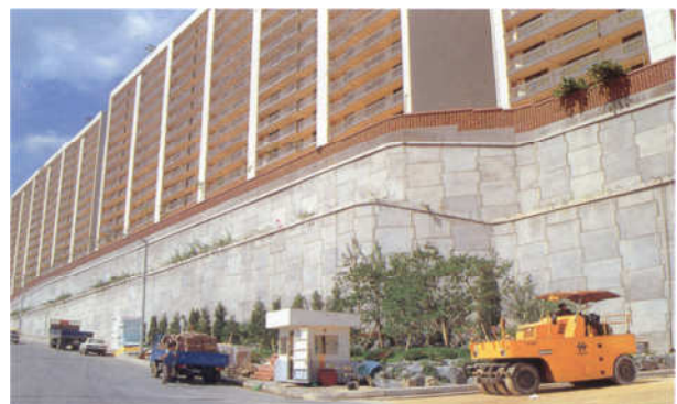
Fig 3.3 Two stages of reinforced wall in Sadangdong, Daelim apartment complex.
