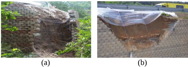
Figure 5.4 Facing wall failure case history (Local road construction area : (a) Deformed of middle part of REW and collapse of facing wall, (b) Facing block sliding)(Lee and Cho, 2011)
