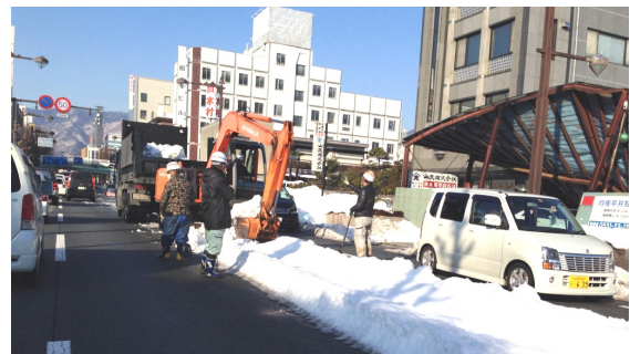
Photo 1 Snow removal using a backhoe
