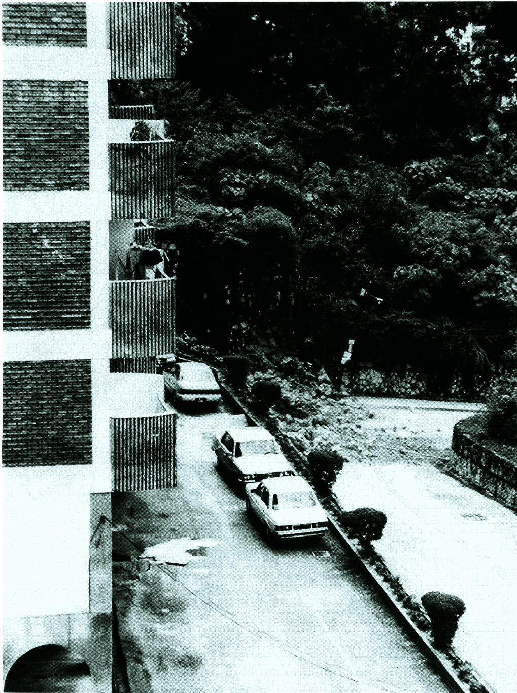
Photo 2 Collapsing retaining wall on side of the building and cracks on parking ground.
