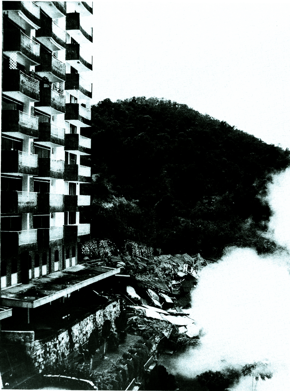
Photo 7 Slid slope and collapsed retaining wall behind the building, 3 minutes after toppling.
