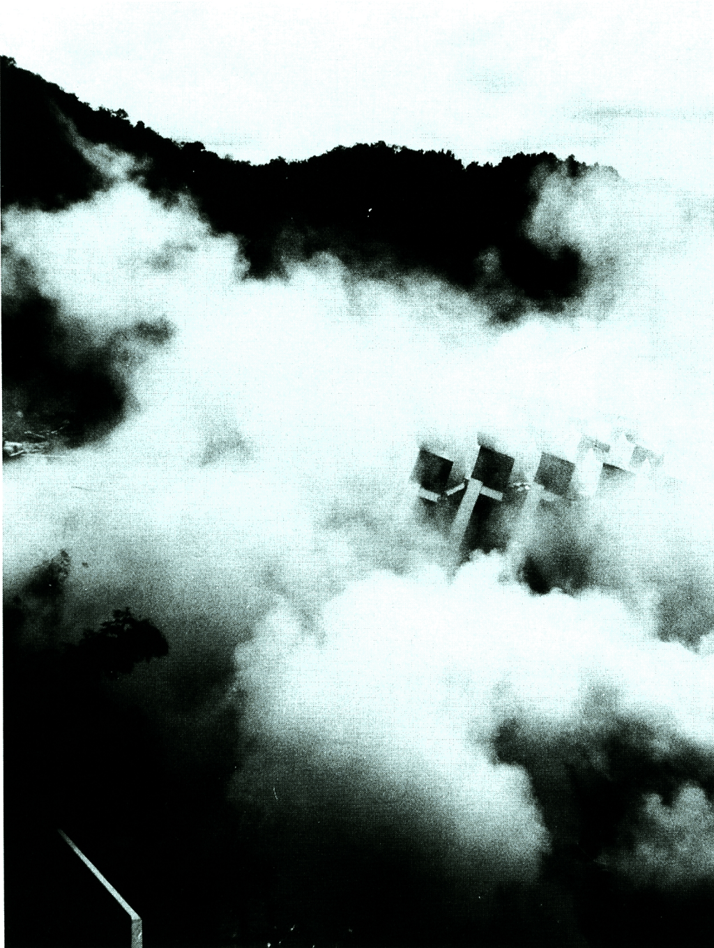
Photo 6 Smoke of the building, 3 minites after toppling.
