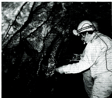
Photo. 1. Headrace tunnel without concrete lining. (Shimo-Nishitani run of the river hydropower station, Chugoku Electric Co. Ltd.)
