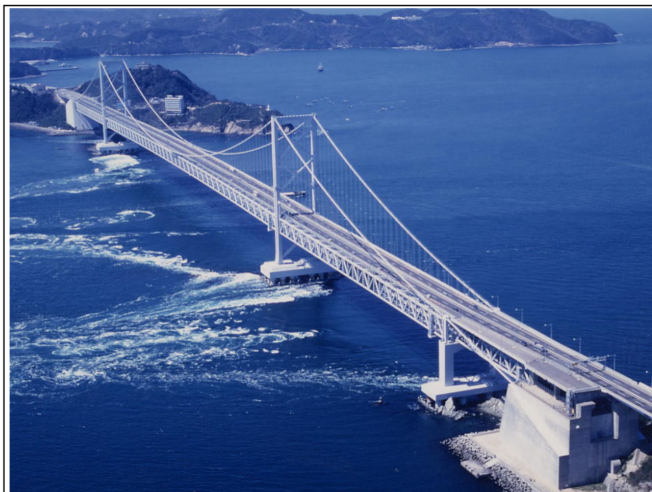
Fig.5.2: The Ohnaruto Bridge, completed in 1985
