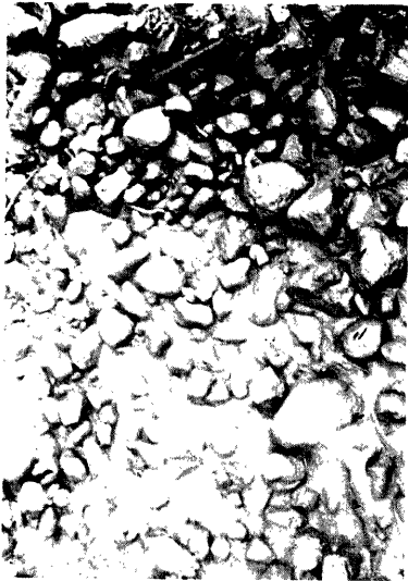
Photo 1-3 5 sec.; the third in the right hand perfectly lacks the matrix in the interstices among the gravels
