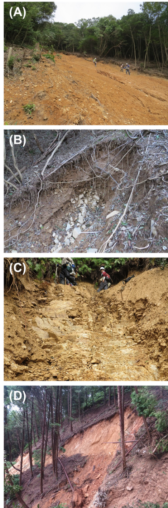
Photo 3 Types of landslides (see Fig. 4 for locations). (A) Planer translational landslide on a granite hillslope. (B) Gash-out failure in a hornfels hillslope. (C) Shallow wedge sliding, and (D) deep, bedrock wedge sliding in the granite area.
