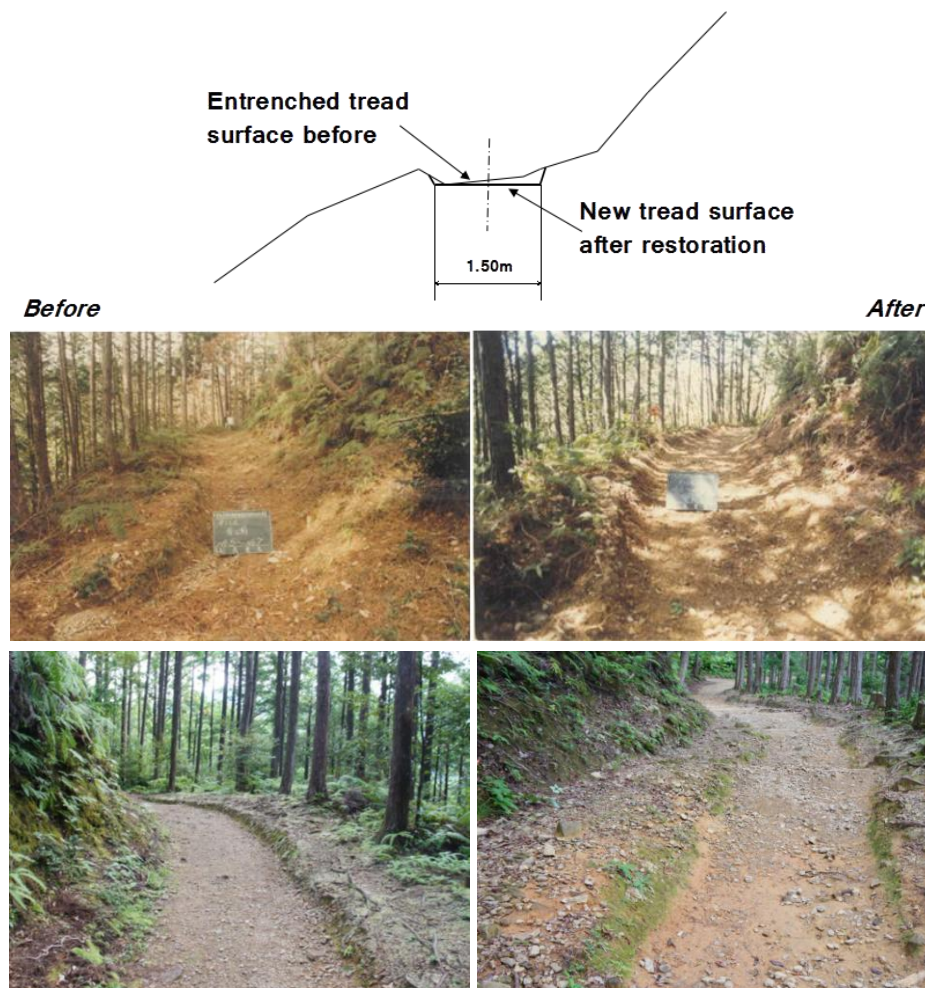
Figure 4.6 An example of the soil excavation practice in the restoration project 1978–1982. a. Upper-left, photo from the construction report that was taken before construction; b. Upper-right, photo from the construction report that was taken after construction. The sketch above the photos was drawn by the author, based on the original design graph (Photos are credited to the Local Education Office of the Hongu-District.). c. Bottom-left, photo taken by the author in 2013 at a location close to the locations of the two photos above. The sharp descent near the trail edge was used for the on-site identification of such practices; d. Bottom-right, a disturbed surface of the entrenched trail caused by lateral erosion. Photo taken by the author in 2013 near that shown in c.
