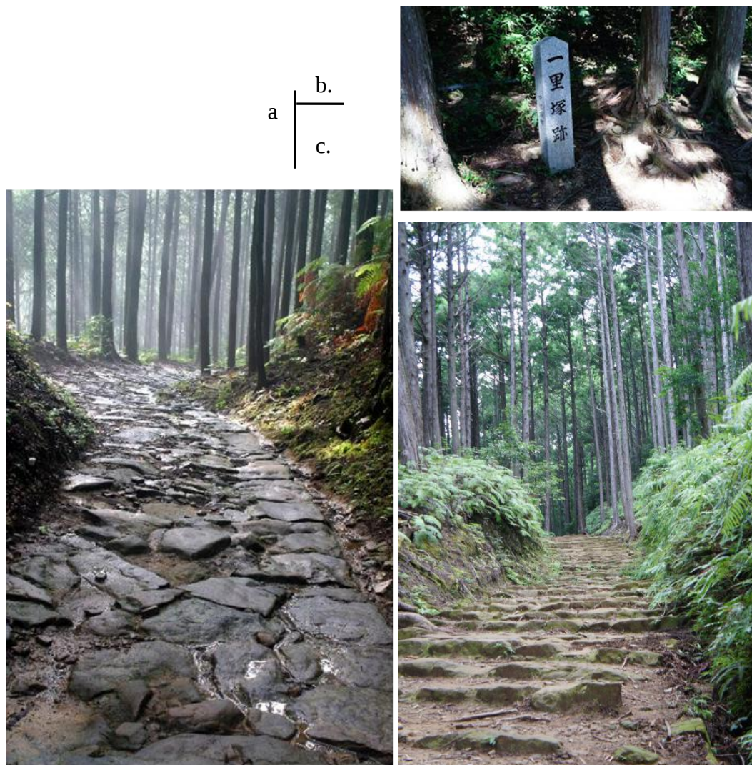
Figure 3.3 Remaining of road reparative and maintaining construction during Edo era ordered by then ruler of the Kishu Domain on Nakahechi Route for the section from Hosshinmon Oji to Kumano Hongu Taisha shrine. a. Stone-pavement; b. Relics of Ichiri zuka (milestone); and c. Stone steps.
