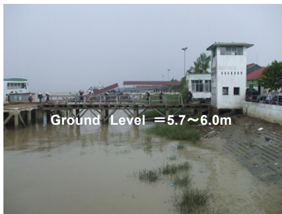
Photo 1 Relation of pier, seawall and road
