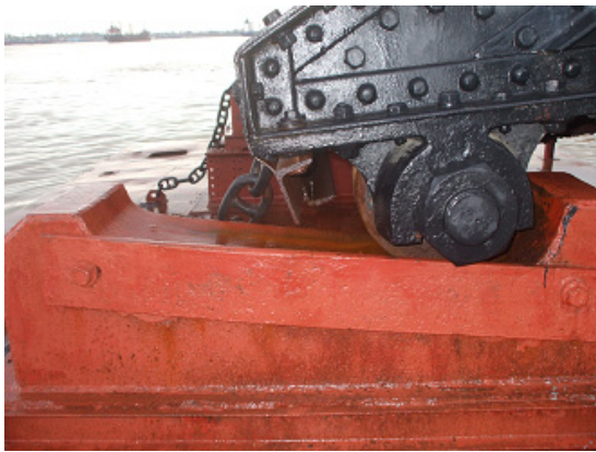
Photo 3 Connection of floating small pontoon and Bridge
