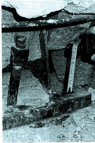
Photo 25 Pull-out of anchor bolts.
