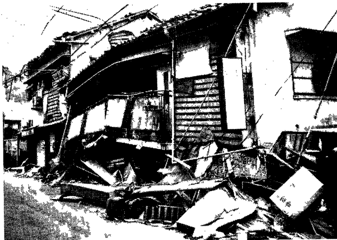
Photo 4 Collapse of wood houses with retail space.
