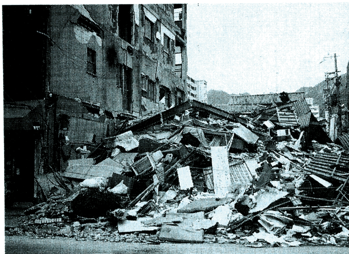
Photo 20 Collapse of 3-story steel structure.
