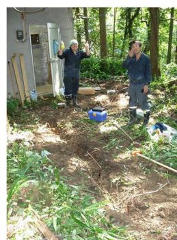
Photo. 7 Class A grounding work
