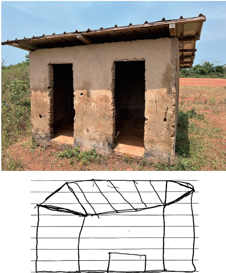
Figure 5 Actual picture (school toilet) and drawing on ideal toilets (Lomie)
