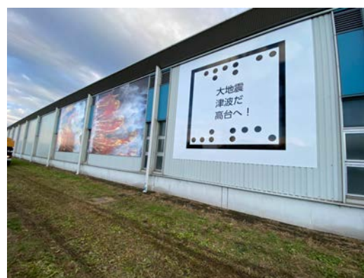
Photo 10 Installed two signboards and one AR signboard
